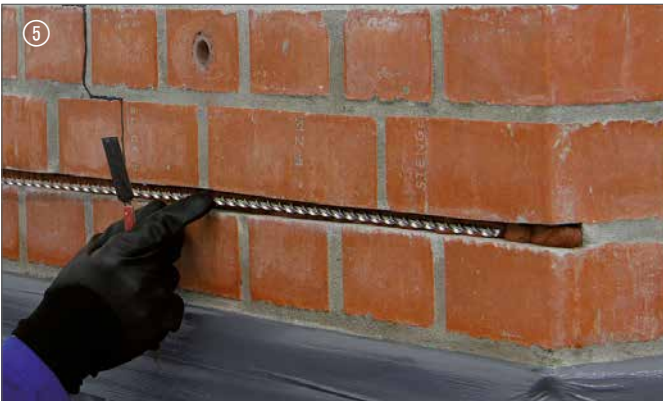
Spiralanker setzen | Place the spiral anchor
