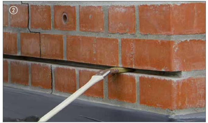
Fuge reinigen | Clean the joint / slot
